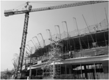
DATA CENTER BANCOMER
